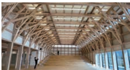
Hall made of domestic Larch LVL, domestic Cypress lumber, and domestic Cypress CLT
