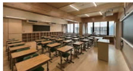
Classroom built with domestic Cedar LVL, domestic Larch LVL, and domestic Cypress CLT
